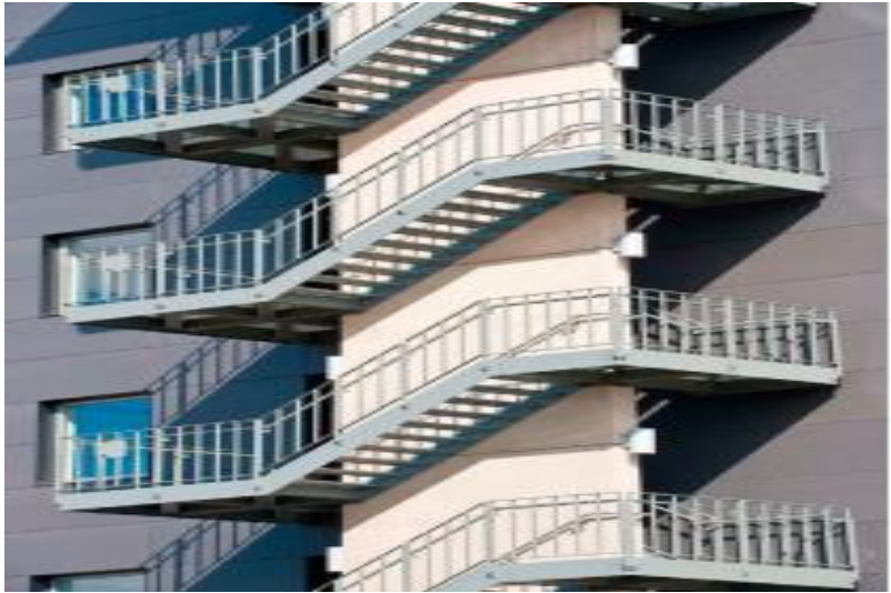
Fig. 10.2. Fire stairs of a multi-storey building
