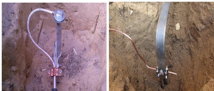
Fig. 5.13. Device trench installation of vertical electrodes
